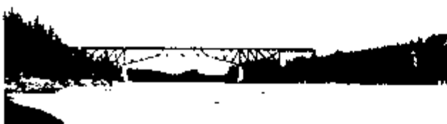
Steel Bridge at Manitou Rapids, c.1920 (courtesy Provincial Archives of Manitoba, John A. Campbell Collection, #189)
