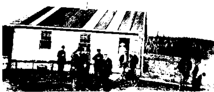
Hudson Bay Construction Office (courtesy Sam Waller Museum, PP 94.2.23a)
