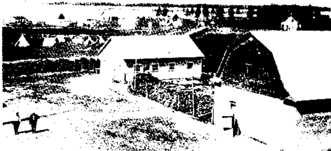
Barn and Shed at Residential School
