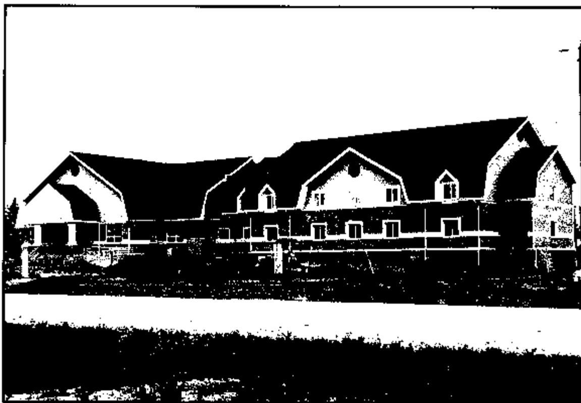
New Hydro Staff House, Grand Rapids, 1997 (Courtesy Lee Heroux)
