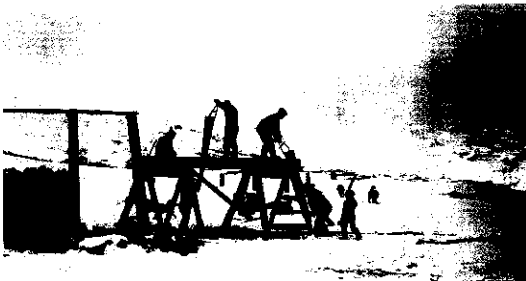
A saw pit cutting logs into boards for houses, N54644 (courtesy National Museums of Canada)
